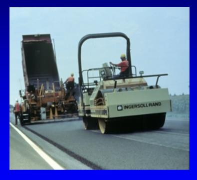
Determine <u>lowest</u> mix laydown temperature that will allow density
