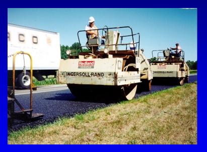
Contractors attempt to extend compaction time - Higher Mix Temperatures - should be LAST RESORT
