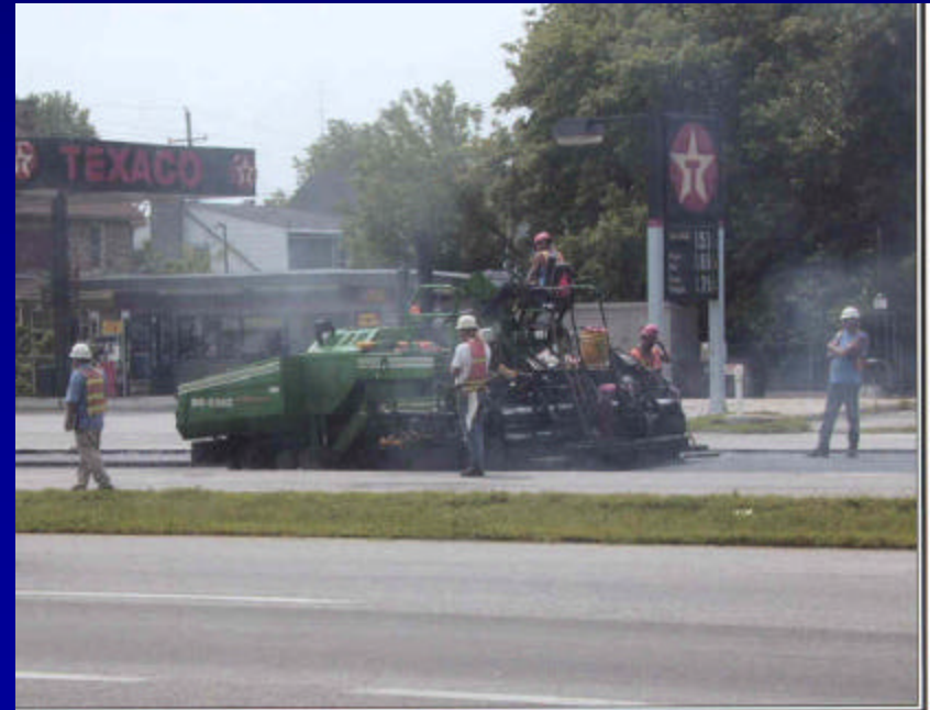
Superpave replaces deteriorated concrete at Landing Road.
