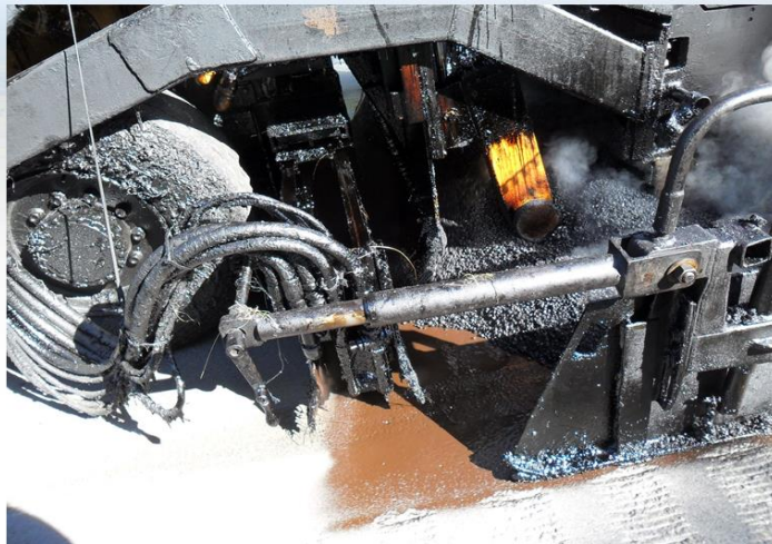
Close up shows the emulsion being spray applied directly before the hot UTBWC material is applied.
