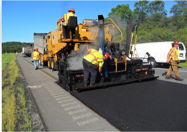
Photo on I-80 of truck dumping plant mix into spray paver and laying hot material directly on emulsion.
