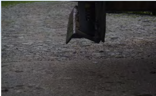
Adjustable Safety Edge Device
