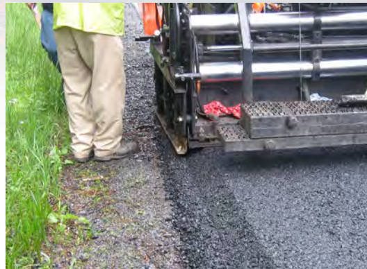
Adjustable Safety Edge Device
