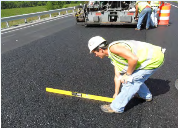
Checking Cross Slope
