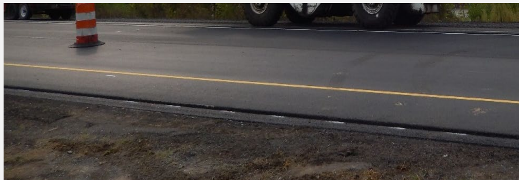
One-inch thick placed 6.3 mm, SR 220
