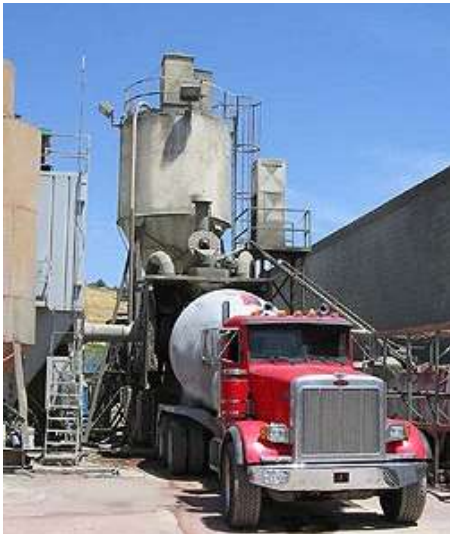
Truck Mixed Concrete
