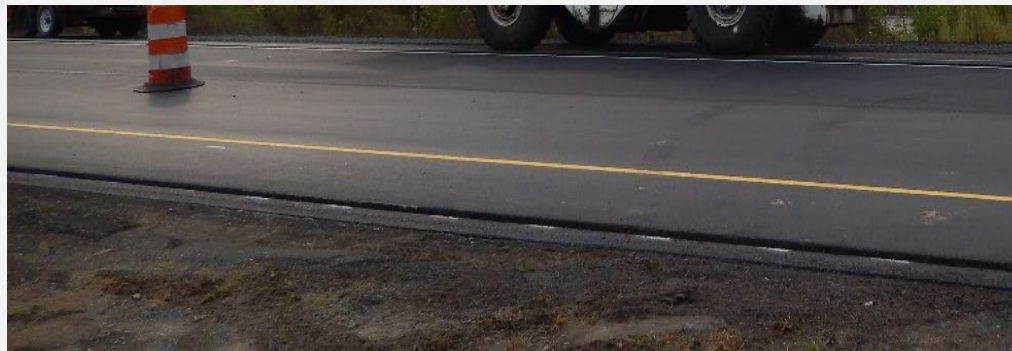
One-inch thick placed 6.3 mm, SR 220
